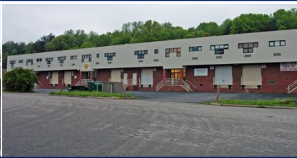
Fullerton Industrial Park 95,000 SF Fairfax County
